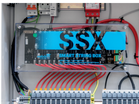
SSX Detail. String box on a photovoltaic plant.
